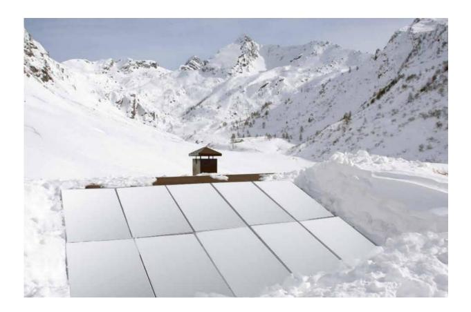
An aluminum plate covers the surface of the snow melting board and the internal insulation heating sheet, which heats up to 80-110 degrees Celsius. Snow and ice can be quickly melted, reducing the damage caused to housing construction.
