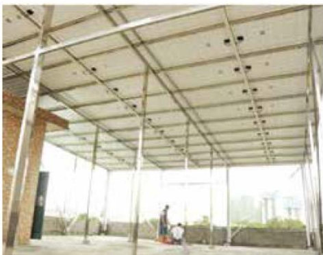
Ground bracket (hot galvanized C-steel)
