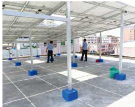
Hot-dip galvanized photovoltaic support
